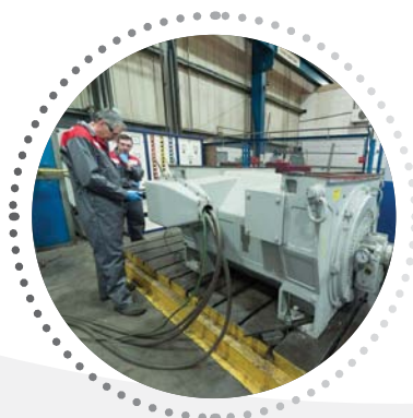
Testing a high voltage motor at our Avonmouth service centre
